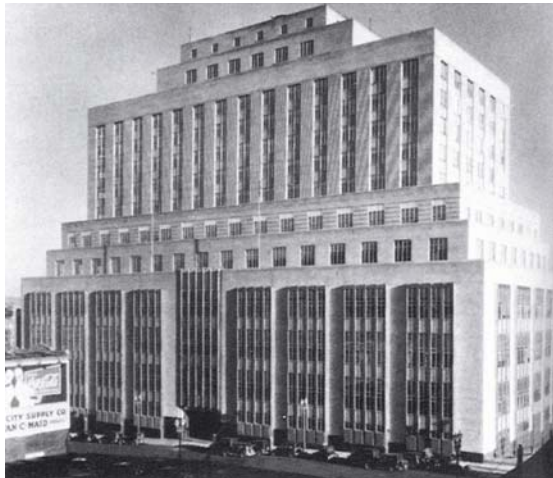
Among the projects that set Kawneer apart was its first curtain wall installation in 1932. The U.S. Post Office in St. Paul, Minnesota was a unique engineering challenge that led to many more successes.
