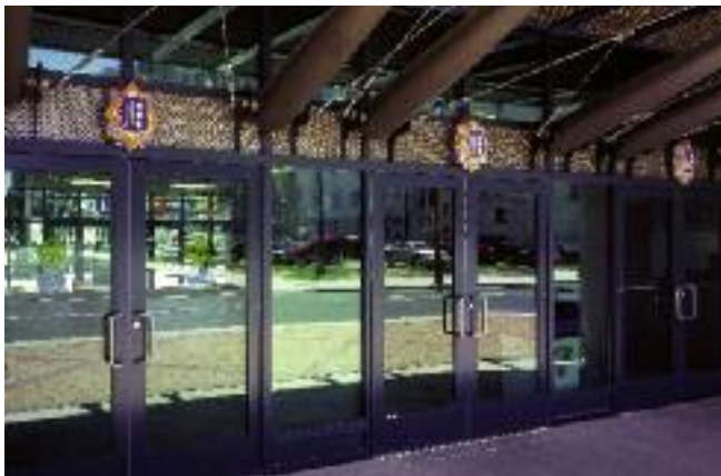
Comerica Park Stadium, Detroit, MI Architects: HOK Sport Facilities Group, Kansas City, MO; Smith, Hinchman and Grylls (SH&G), Detroit, MI; Rockwell Group, New York, NY Glazing Contractor: Universal Glass & Metals, Inc., Detroit, MI
