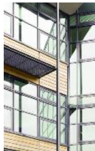
Peninsula Medical School, Plymouth, United Kingdom Architect: Nightingale Associates, Oxford, United Kingdom Glazing Contractor: Dudley's Architectural Aluminum, Cardiff, United Kingdom
