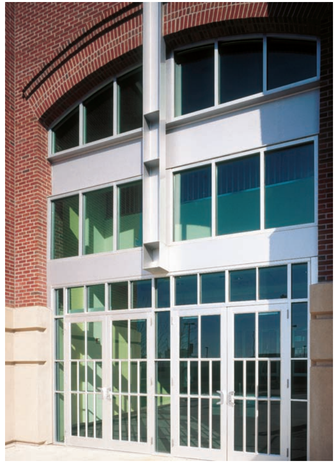
Baltimore Ravens Stadium at Camden Yards, Baltimore, MD Architects: Hok Sport Facilities Group, Kansas City, MO; Robert P. Madison International, Inc., Dallas, TX Glazing Contractor: Zephyr Aluminum, Inc., Timonium, MD
