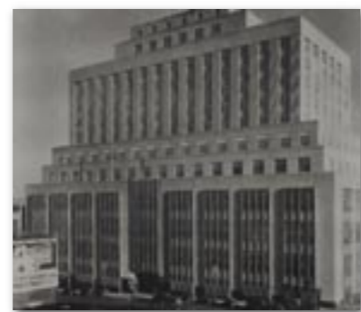
Aluminum Curtain Wall 1930
