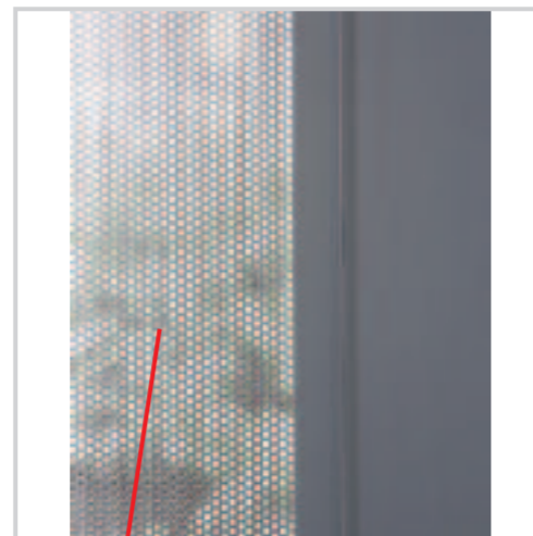
Perforated stainless steel mesh offers ventilation and visibility (as shown in 'Security Level 3' pictures on page 9)
