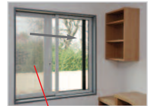
Mesh comes across the window on opening allowing good visibility but preventing the flow of contraband in or out of the window
