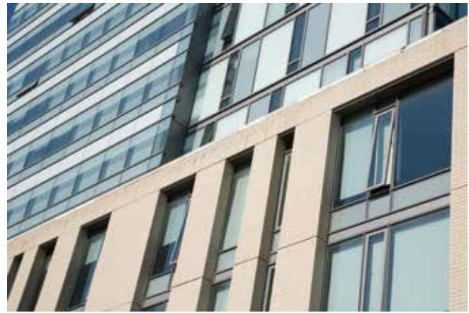
Woodsworth College Residence, University of Toronto, Toronto, Ontario, Canada Architect: architectsAlliance, Toronto, Ontario, Canada Glazing Contractor: Ferguson-Neudorf Glass, Inc., Beamsville, Ontario, Canada
